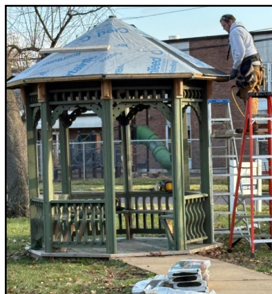
A worker with Agape Construction lays shingles on the roof.
